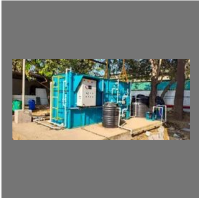
Sewage Water Treatment Plant
