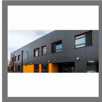
Exterior ACP Cladding
