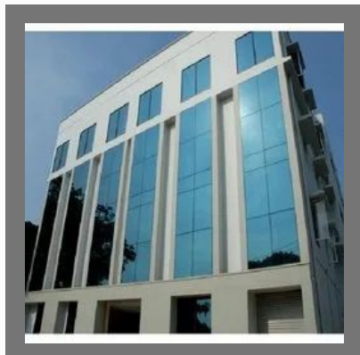
Structural Glass Glazing Work
