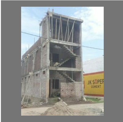
Building Construction With Material
