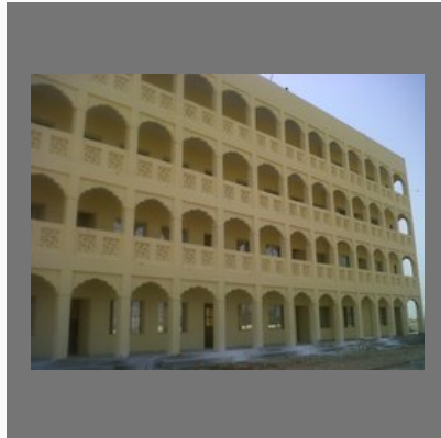
School Building Construction
