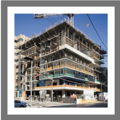
Commercial Buildings Construction Service
