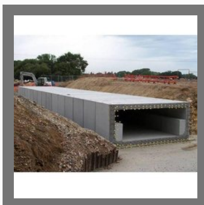
Culverts Construction Service
