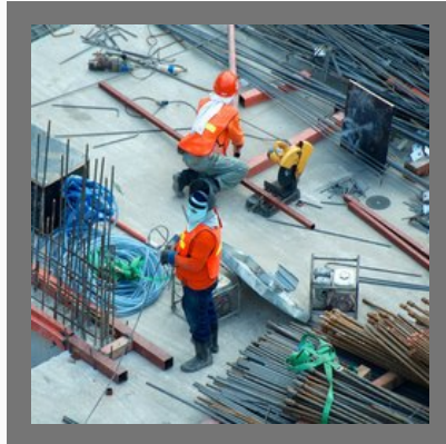
Commercial Construction Service
