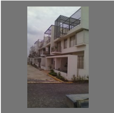
House Construction Service
