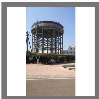
Water Tank Construction Service
