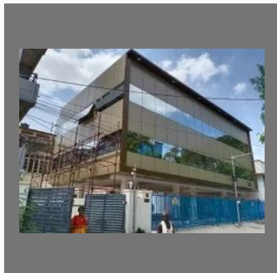
ACP Elevation Work
