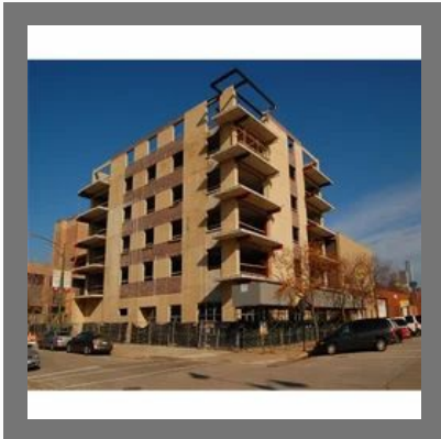
Industrial Building Construction
