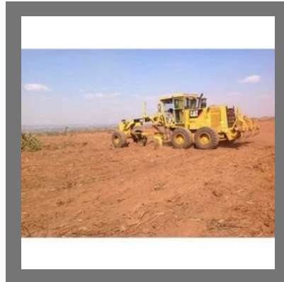
Land Leveling Work
