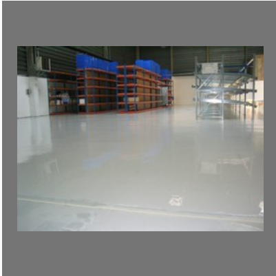
Epoxy Self Leveling
