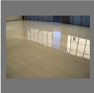
Epoxy Floor Coating Services
