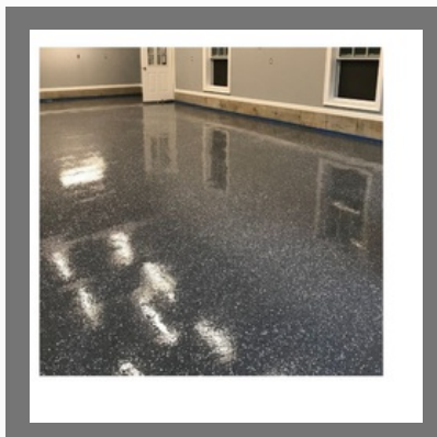
Epoxy Floor Coatings
