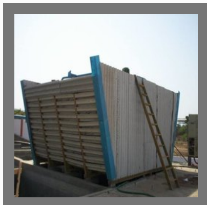
Wooden Cooling Tower
