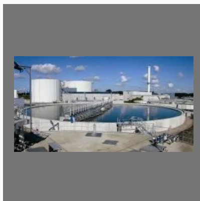
Effluent Treatment System
