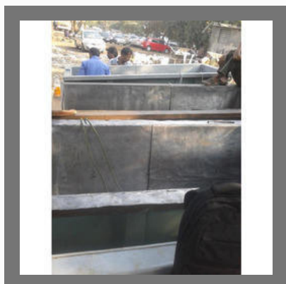
Lead Lining Tanks
