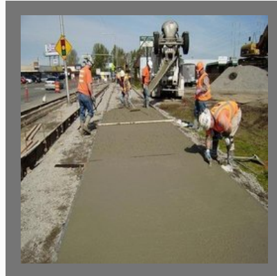
C C Road Construction Services
