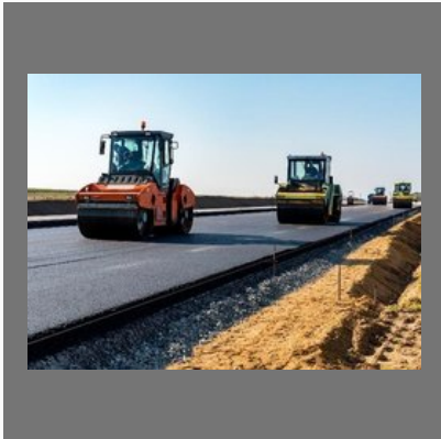
Bitumen Road Construction Contract Services
