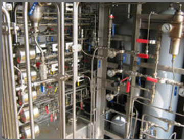
Fabrication And Erection Of Equipments
