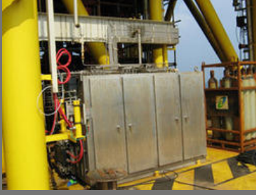
Heavy Equipments Erections And Commissioning
