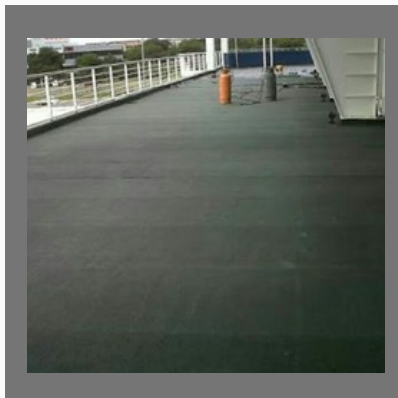
Water Based Epoxy Coating
