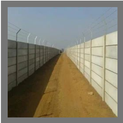
RCC Compound Wall
