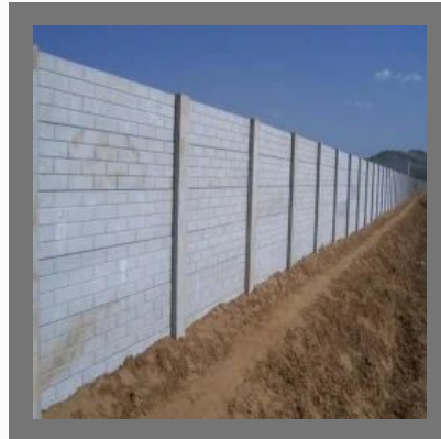
Brick Pattern RCC Compound Wall
