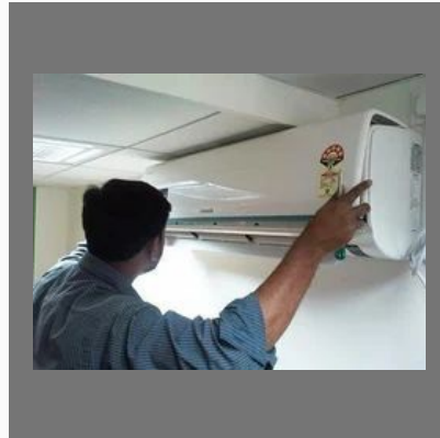
Air Conditioner Repairing Services
