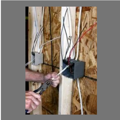
Residential Electrical Contractor
