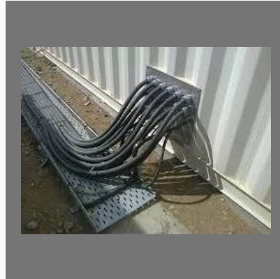
LT Cable Laying
