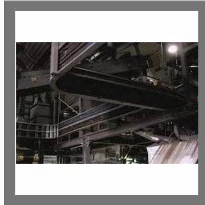
Cable Tray Installation Services
