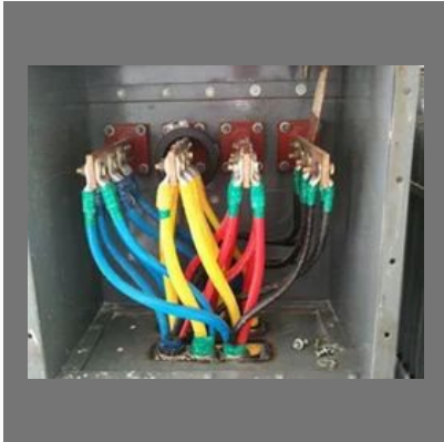
LT Cable Laying and Termination
