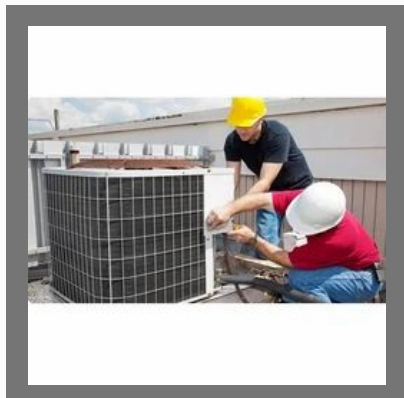
AC Installation Services
