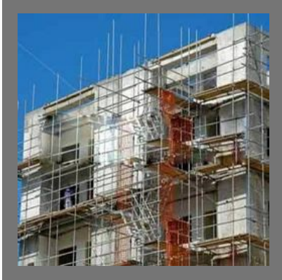
Residential Apartment Construction Services
