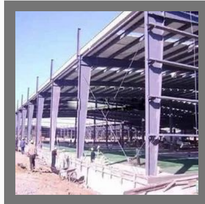
Factory Buildings Construction Services
