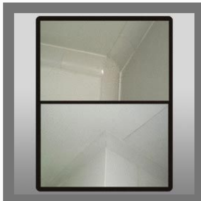
Clean Room Covings
