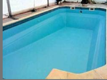
FRP Lining Work on RCC
