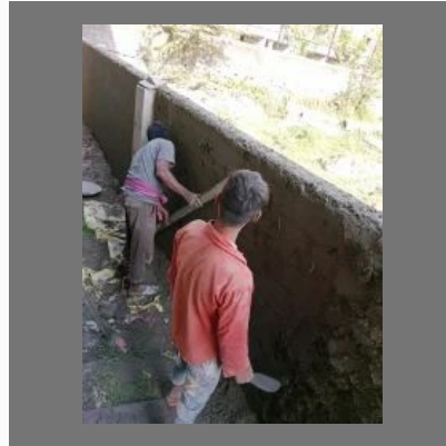
Boundary Wall Construction Work
