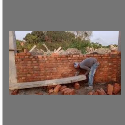
Commercial Building Construction Work
