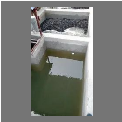
Concrete Water Tank
