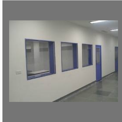
Doors and View Panels
