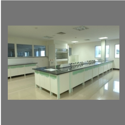
Fume Hood & Lab Furniture
