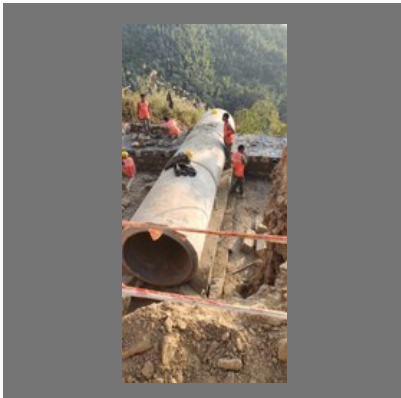
Water Pipe Line Works
