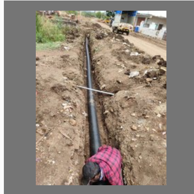
Pipe Line Work
