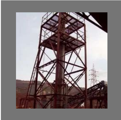
Column Flotation cell
