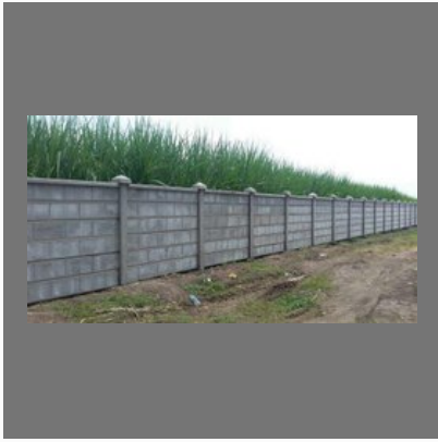
Precast Boundary Wall
