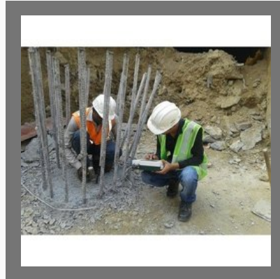
Pile Integrity Testing Services
