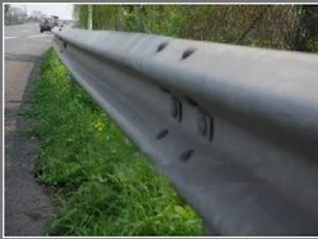
Steel Crash Barrier
