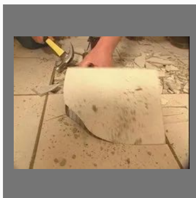
Floor Tile Demolition Service
