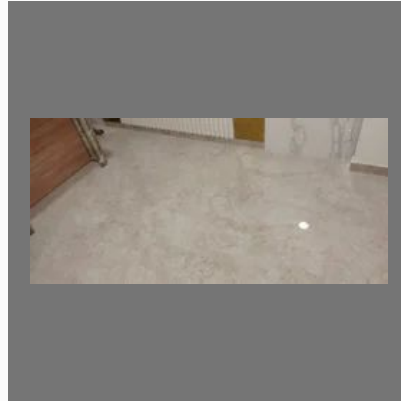
floor tiles fixing Tata Croma side
