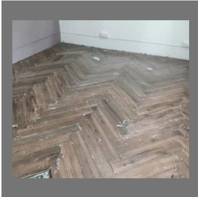
Wooden Floor Tiles Installation Service
