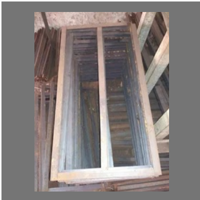
H Frames Scaffolding
