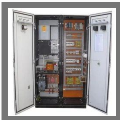
Schneider VFD Control Panel Service
