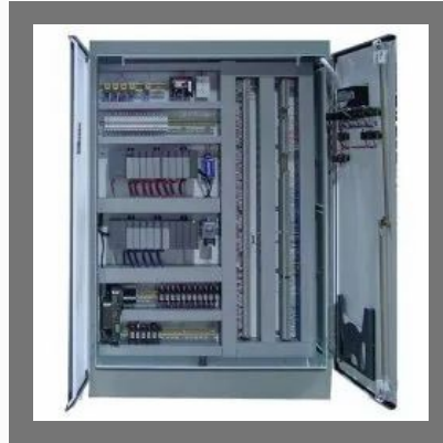
Plc Control Panel Repairing And Service
