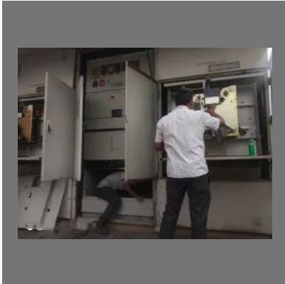
Vcb Repairing And Services
