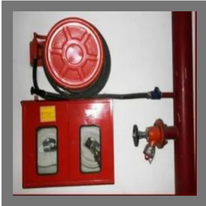
Fire Hydrant Installation
