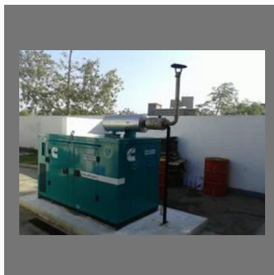
DG Set Repairing Service
