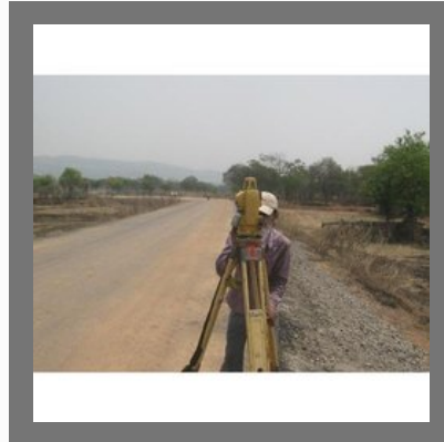
Alignment Survey Services
