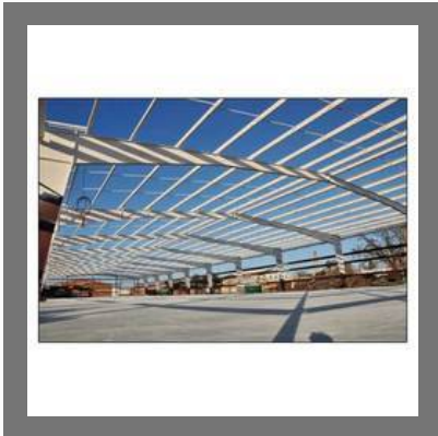
Pre Engineered Metal Building
