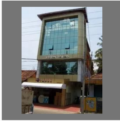
acp cladding and glazing
