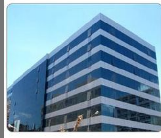
Structural Glazing Work
