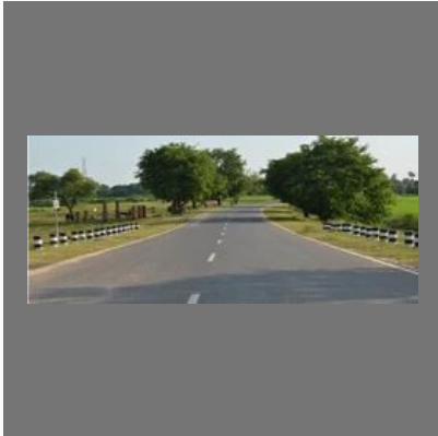
Highway Road Construction
