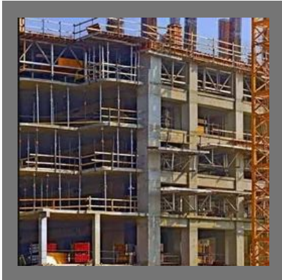
Residential Building Construction
