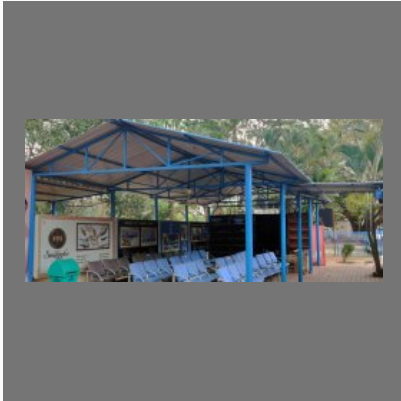
Mild Steel PEB Structural Shed
