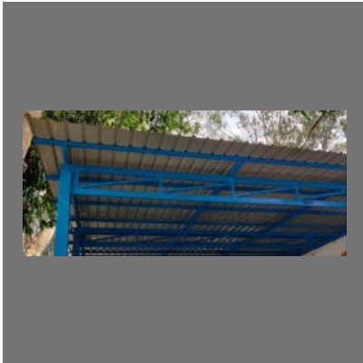
Mild Steel Structural Factory Roofing Shed
