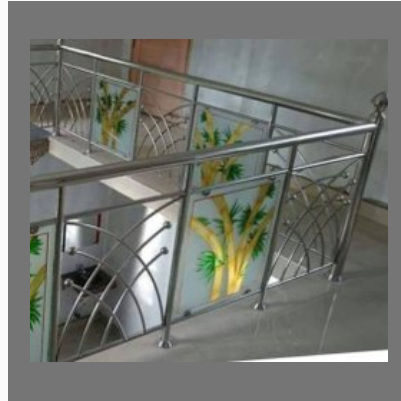
Ss Balcony Glass Railing
