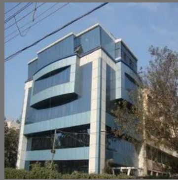
Commercial Office Construction Service
