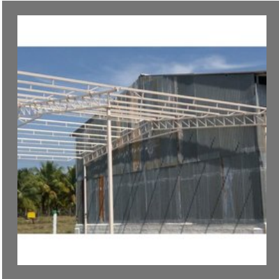
Pre Engineering Building
