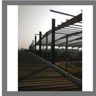
Pre Structural Building
