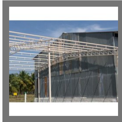
Pre Engineering Building
