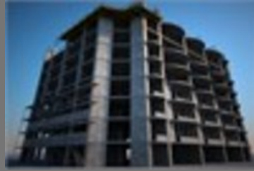
Building Construction Services
