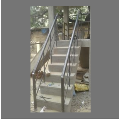
Mild Steel Stair Railing
