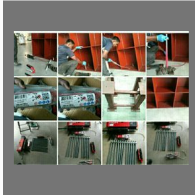
Hilti Chemical Bolt Fixing Services
