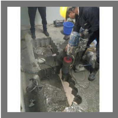
RCC Cutting Services
