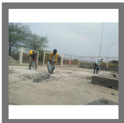
Commercial Concrete Breaking Services
