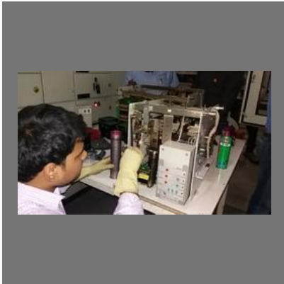
Breaker Repairing Services
