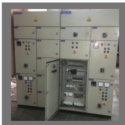
Main LT Panel With Load Management (LMS)
