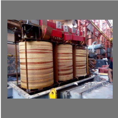
Transformer Repairing Services
