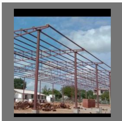
Roofing Shed Structures
