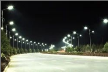
Street Light Maintenance
