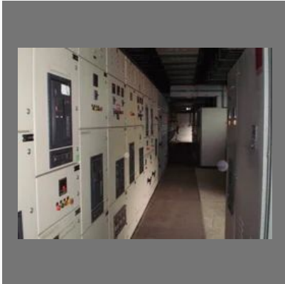
Testing & Commissioning of Panel Boards
