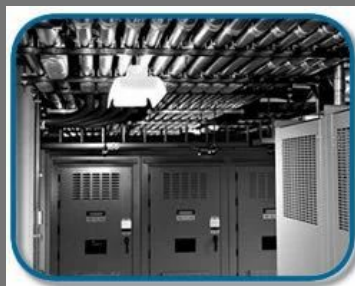
Laying Of Low Tension Cables
