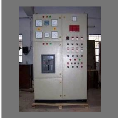
Erection of AMF Panels
