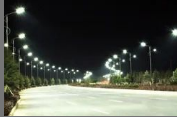
Street Light Erection
