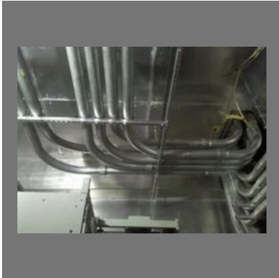
Erection of MS Conduit Wiring System
