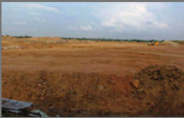
Office Building Construction Services
