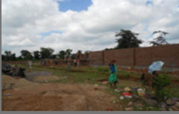
School Building Construction Services
