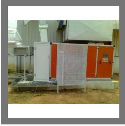
Industrial AC Repairing Service
