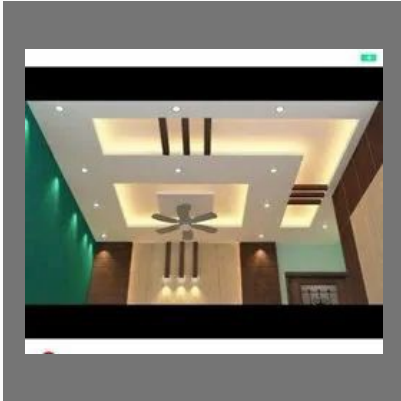
Office False Ceiling Service
