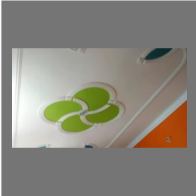
Bedroom False Ceiling Work
