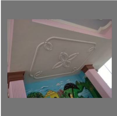
Bedroom False Ceiling Work
