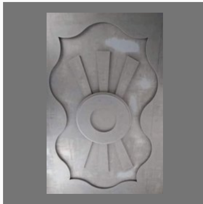
POP False Ceiling Work
